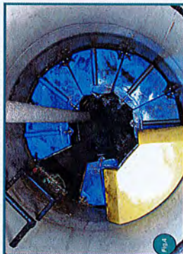
Compliance with your stormwater treatment permit requires using suitable Up-Flo® filter replacement media bags from Hydro International to ensure the system is functioning as intended (Fig. 2)
